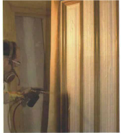
Accent color on doors. Armed with plenty of masking tape, and a steady hand with an X-acto knife, one of the authors masks off areas that don't get a second color, then applies a wiping stain to what's left.
